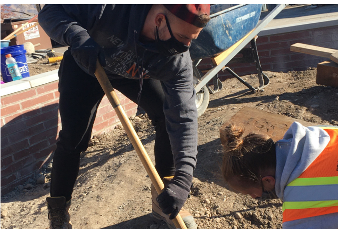
Brandon Thomas backfilling along new gabion retaining walls.
